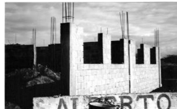
The new worship center is well under way. The walls for the first floor are up, and the dirt has been leveled. Now, they are ready to lay rebar and pour concrete for the floors.
