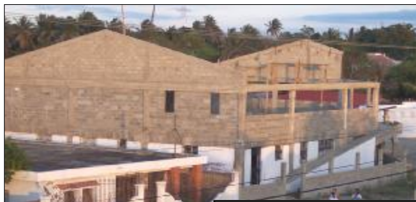
Ready for the Roof
